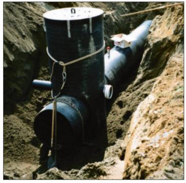
remediation costs, use native material for backfill and maintain the same flow as 36" concrete pipe while maximizing ground cover. Based on the significant savings in material and installation, the district is now considering using HDPE pipe in an increasing number
